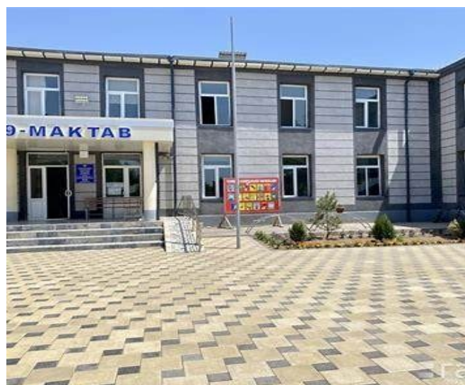
Fig. 6 b) School No. 19 (mahalla "Iftikhor", Bayavut, Syrdarya region): heating on heat pumps, 3×HP, total 340 kW
