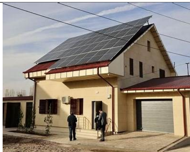
Fig. 6 a) Demonstration energy-saving residential building of the "Near Zero Energy" type (Yoshlik mahalla, Nurafshan city, Tashkent region): a 16 kW solar power plant and solar collectors for hot water supply are located on the roof; heating/cooling is implemented using a heat pump.
